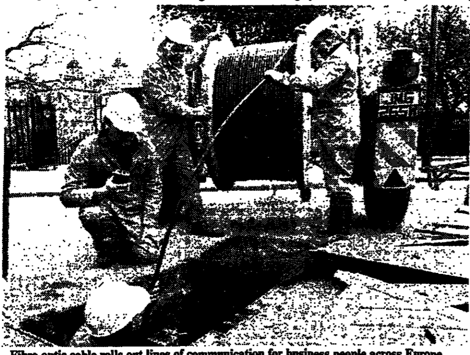
Fibre-optic cable rolls out lines of communication for business people across Europe
